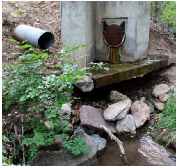
Figure 2.7: Storm drain outfall into Red Butte Creek in Research Park
